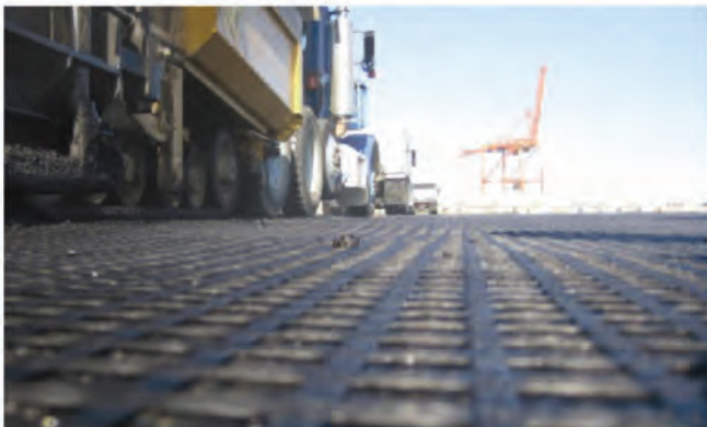
← Port of Seattle Terminal 10 Project Uses Checkmate's Roadgrid Pavement Reinforcement Geogrid
