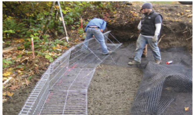
King County Stream 5 Pedestrian Project Uses → Checkmate's Posilok MSE Wall System
